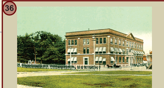
36 Building 86 US Navy converted the second floor of this building into negotiation rooms where the Treaty was formally negotiated and signed on September 5, 1905 at 3:47 pm.
